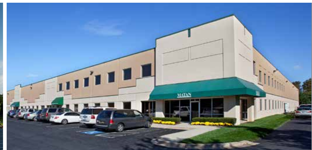
Matan Headquarters Wedgewood II
