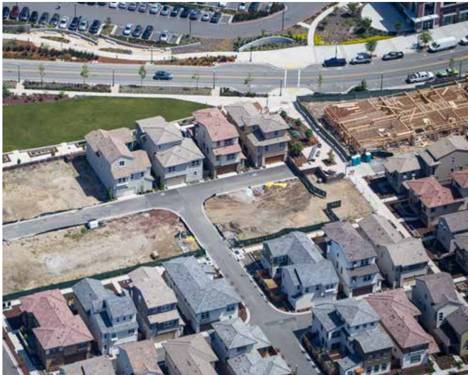
Phase II Under Construction
