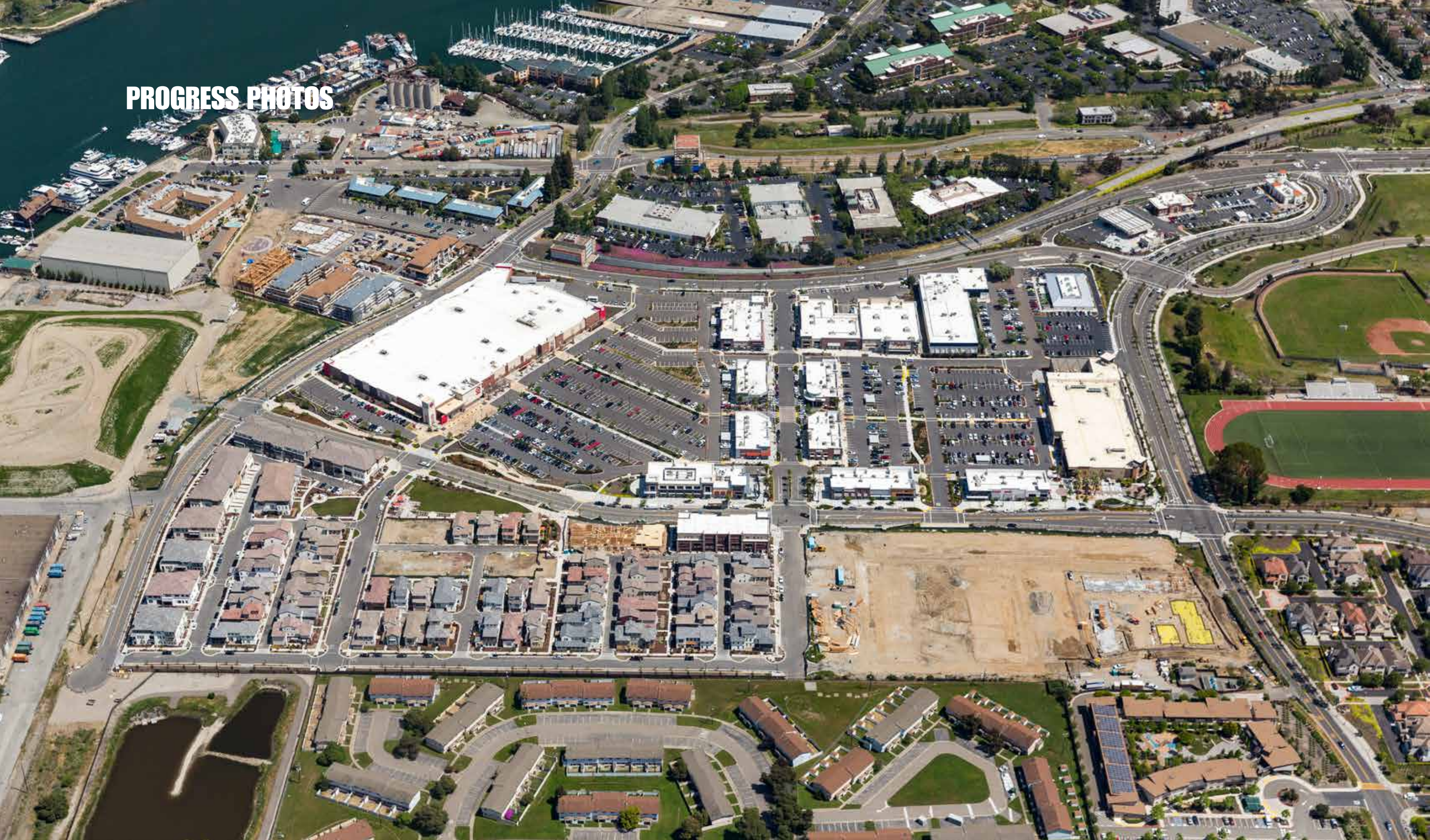
Alameda Landing Shopping Center is almost complete! The aerial view of the community, looking north toward the Oakland Estuary, shows the construction progress.
